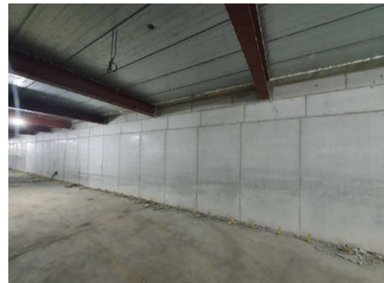
Fig. 13 High Quality Outer Wall after Form Striking
