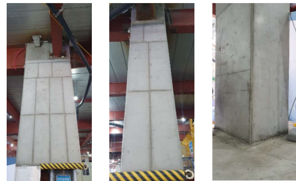
Fig. 12 High Surface Quality of Column using SCC
