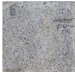
Rough surface (Jet chisel)
