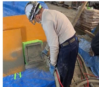
Fig.4 Casting of the second layer by shotcrete method
