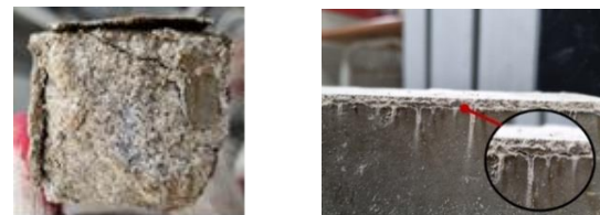
(a) Surface destruction (b) Surface separation Fig.6 Changes in the surface state of specimen (C-SCG)
