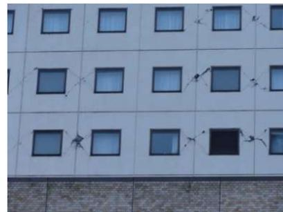
**Fig.1** Damage of non-structural walls observed in the 2016 Kumamoto earthquake
