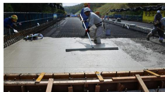
Fig. 1(c) Placing of highly durable concrete
