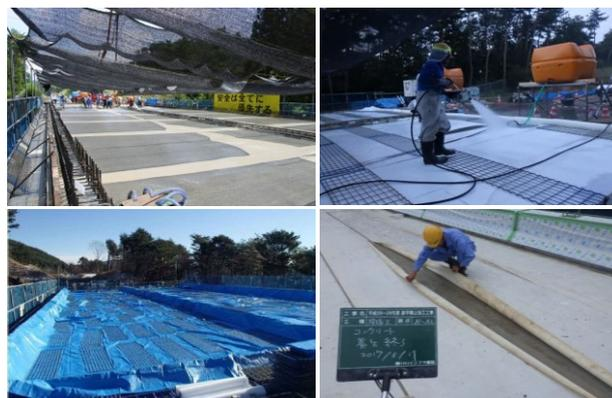
Fig. 1(b) Curing methods adopted for the deck slab
