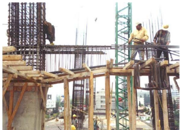
Fig. 1 RC building with haunched beams constructed in Mexico City
