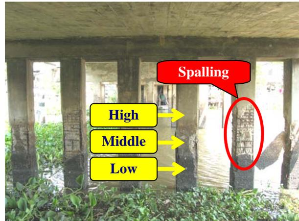
Fig.3 Example of deterioration condition and location of collecting concrete powder sample
