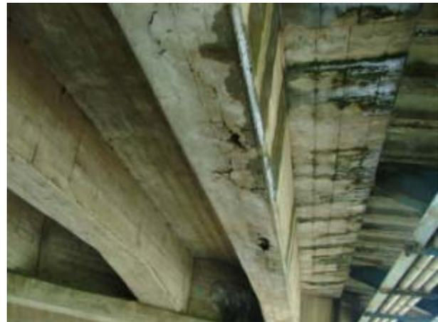
Fig. 7 Main girder deterioration
